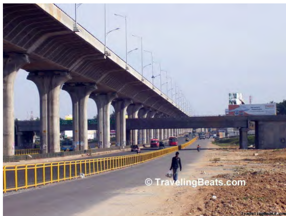
Box-Girder Type Expressway with Single Pier
