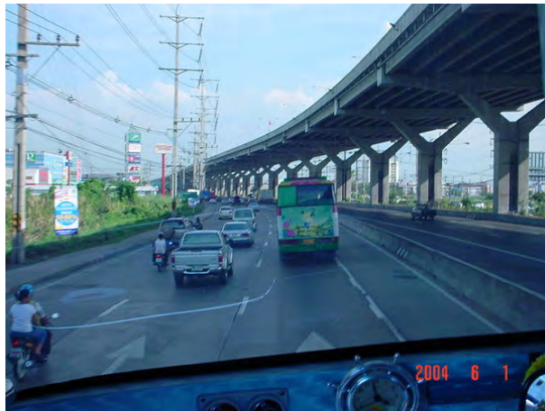
I-Girder Type Expressway with Single Pier
