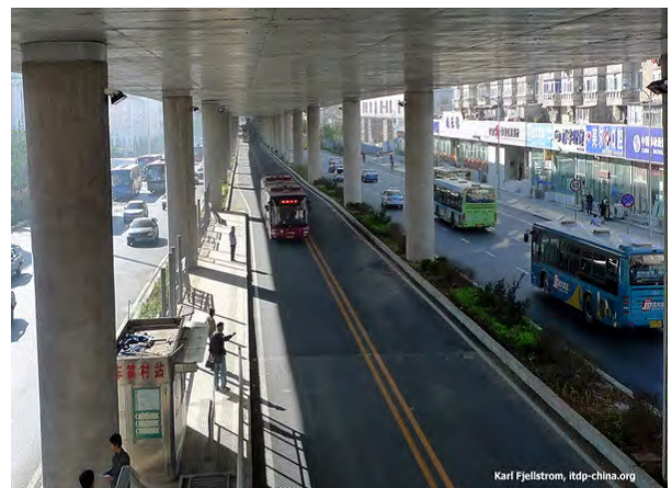
Box-Girder Type Expressway with Portal Frame
