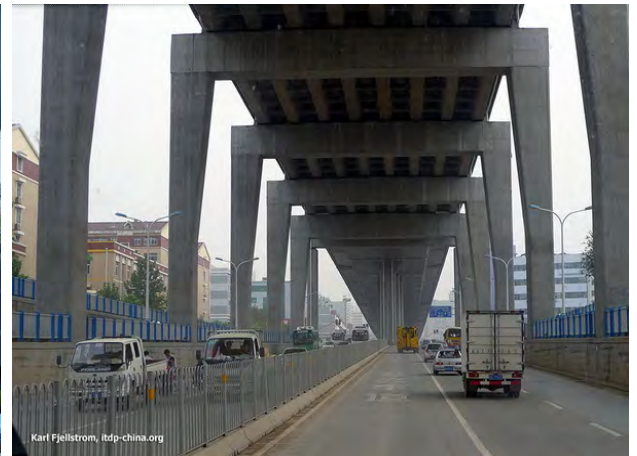
I-Girder Type Expressway with Portal Frame
